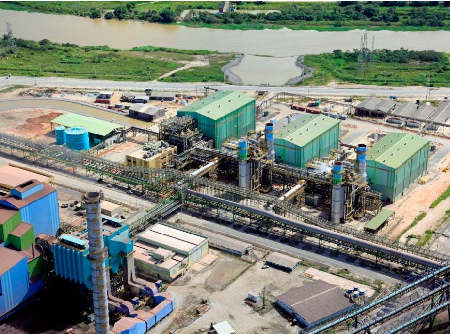
Atlantic Steel power plant, Sepetiba, Brazil
