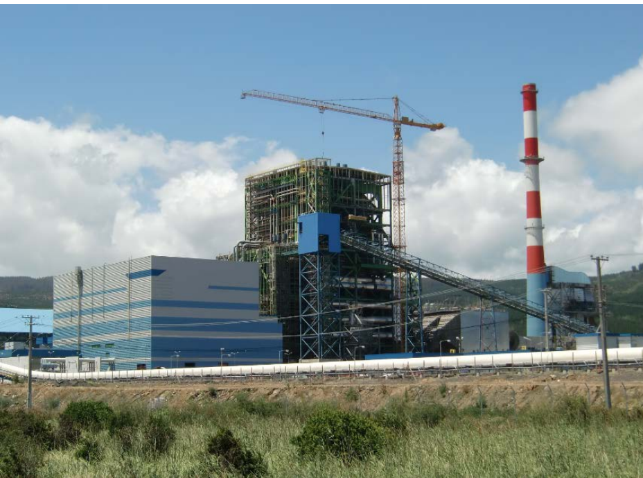
St. Maria I coal-fired power plant in Coronel, Chile (construction phase)
