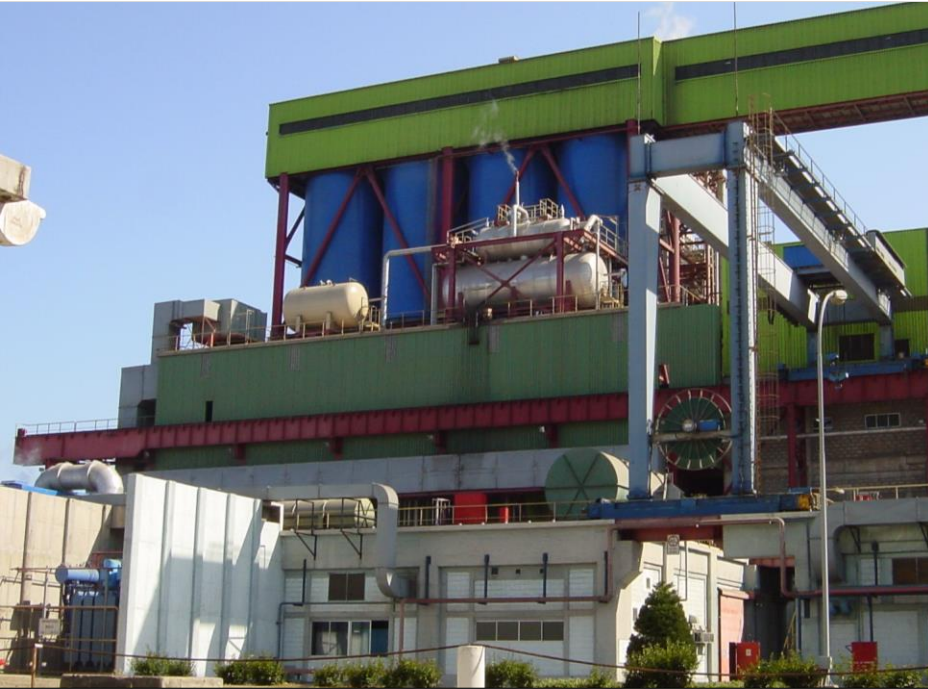
Power plant Guacolda
