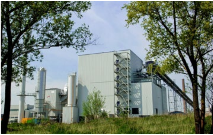
Waste wood utilization at the biomass power plant Lünen
